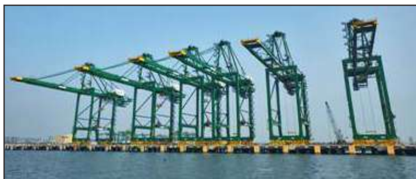
Fourth Container Terminal at JNPT
