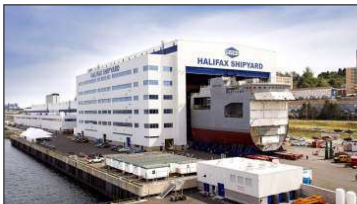
The second mega-block emerges from the Halifax Shipyard's Ultra Hall ... and
