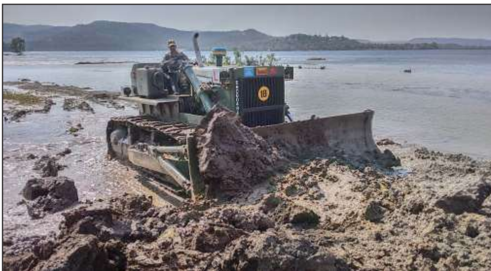
Earth Mover in action on the shores of Khadakwasla Lake
